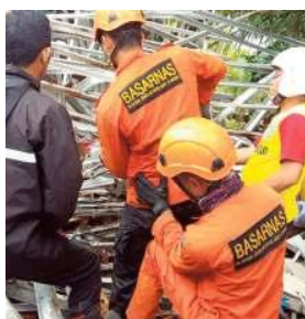
Debris being cleared after a tsunami hits Banten province, Indonesia.
